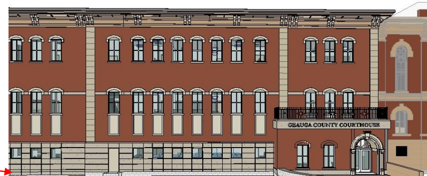
View from 2 nd floor of Annex building across the street from addition – rooftop mechanical unit not visible
